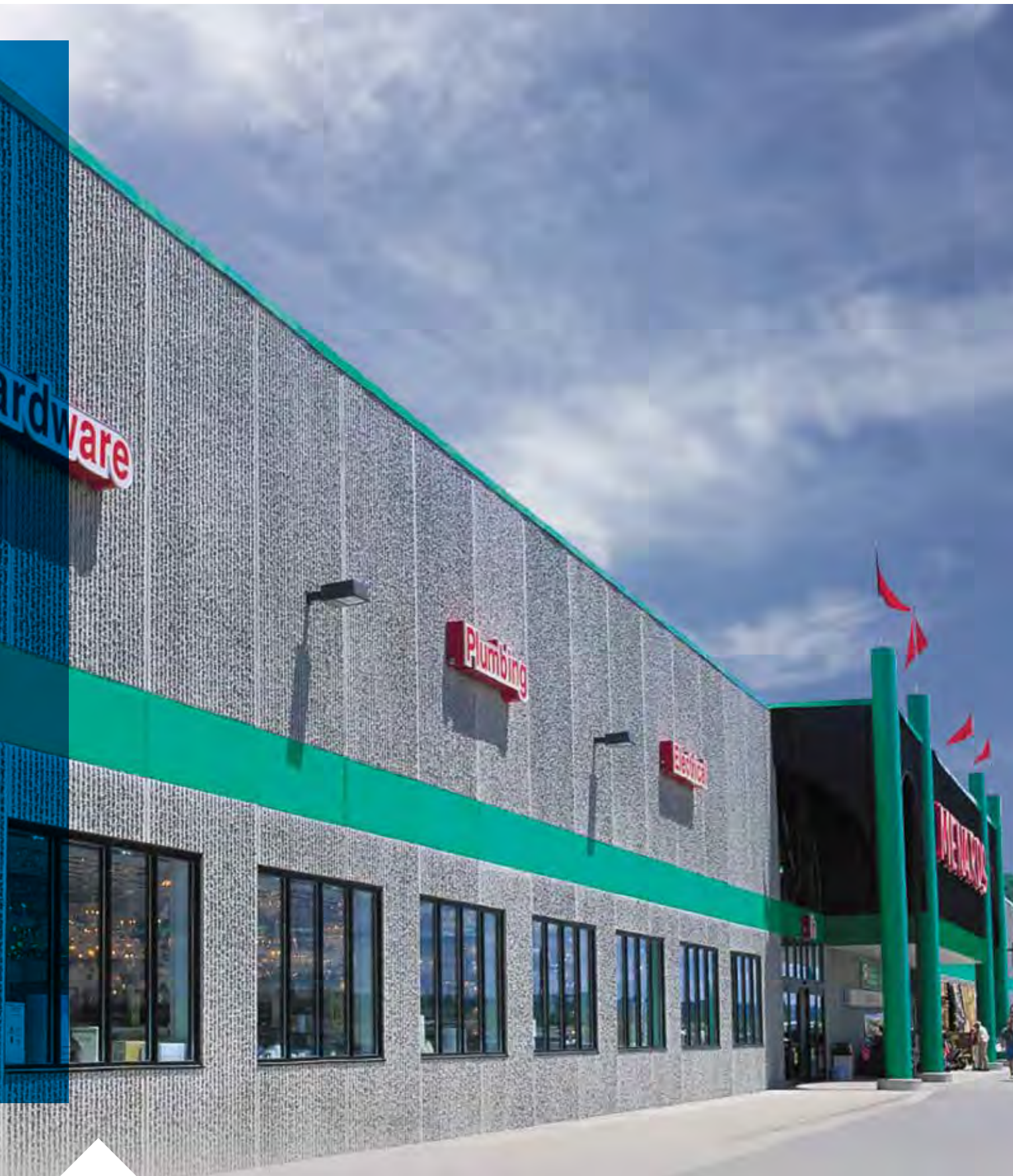
Menards – Wide Rake, Troweled Band (Painted)
