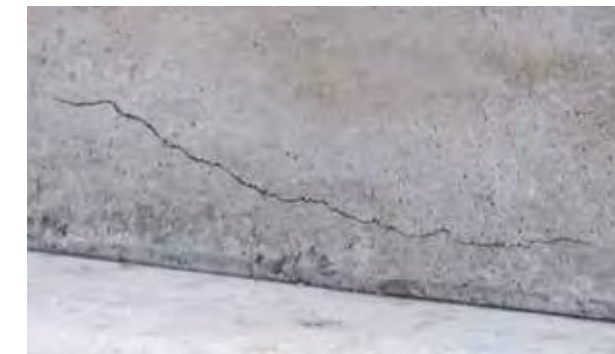
SIDEFORM CRACKS
