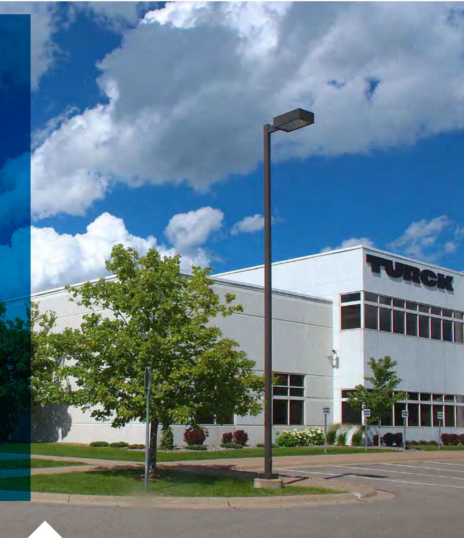
Turck – Formside Exposed Aggregate with Non-Exposed Reveals, White Silica Sand and 100% White Cement
