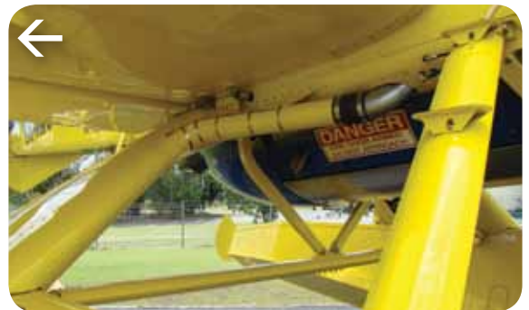
Plate 16. Shows the transfer plumbing from the scoops to the hopper of the Fire Boss.
