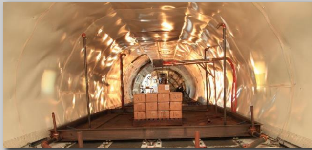
Full-Scale Test (Before)
