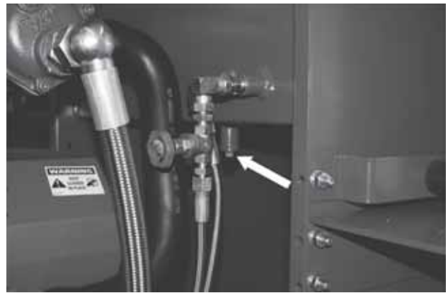
Fig. 36 Drain plug on the fuel tank
