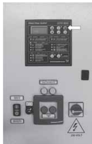
Fig. 32 Manual resetting of alarms
