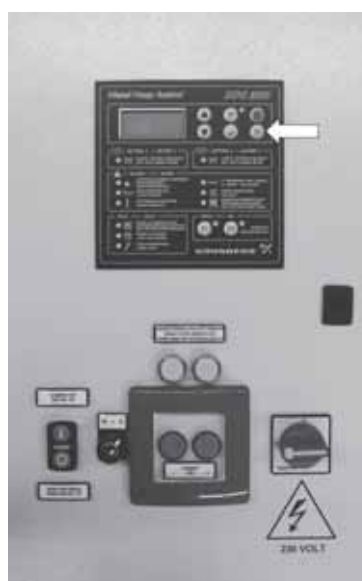
Fig. 46 Indicator light test
