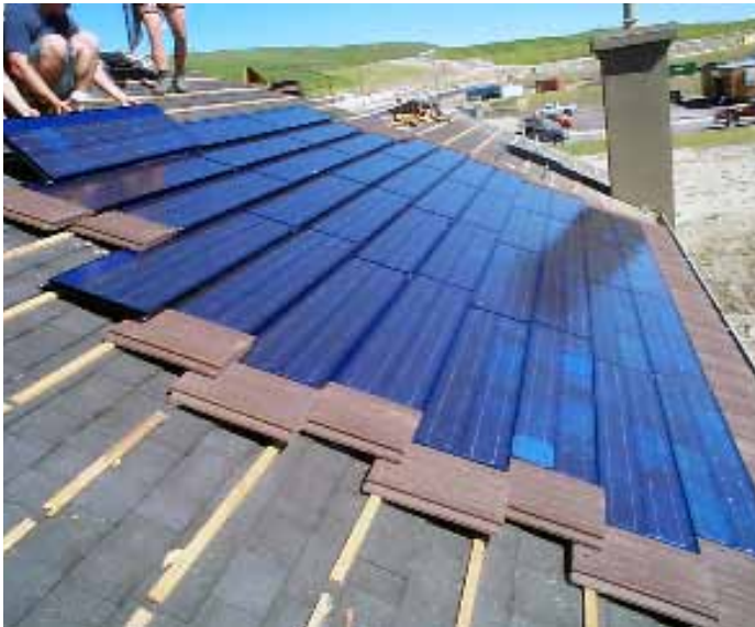
Installation of roof integrated PV system.
