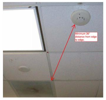
5. Smoke detectors must be spaced in accordance with NFPA 72 and manufacturer's specifications. Refer to NFPA 72 Annex B for design criteria for unique spaces, including those with ceilings higher than 16 feet.
