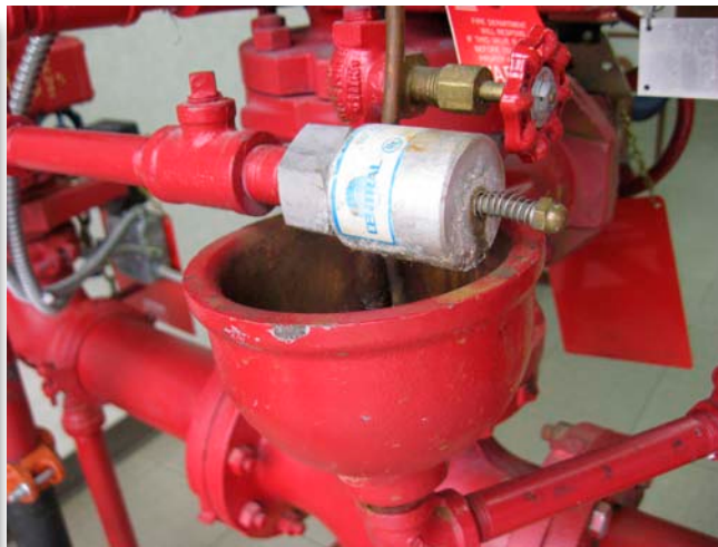
Photo 5: Velocity Drip Drain. The plunger extends out of the housing and is spring-loaded. Corrosion can accumulate inside this device and prevent it from properly draining. This is the plunger that may be depressed when testing the waterflow alarm. In the event the check valve does not seat fully, water will enter into the intermediate chamber trim piping. If the velocity drip drain is also plugged with corrosion, the valve may trip.
