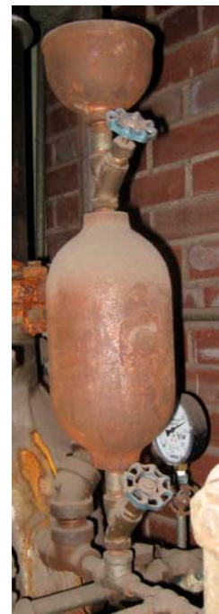
Photo 5: Velocity Drip Drain. The plunger extends out of the housing and is spring-loaded. Corrosion can accumulate inside this device and prevent it from properly draining. This is the plunger that may be depressed when testing the waterflow alarm. In the event the check valve does not seat fully, water will enter into the intermediate chamber trim piping. If the velocity drip drain is also plugged with corrosion, the valve may trip.
