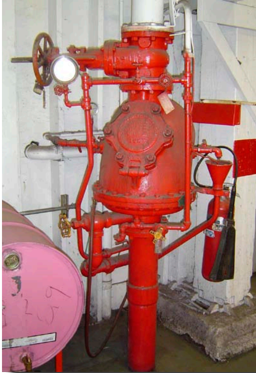
Photo 2: 1922 Rockwood Model A dry pipe valve, which is still in service. Originally developed in 1908 and improved in 1909, the large bulge in the rear of the valve is for a counterweight arm that helps raise the clapper when the valve trips. The clapper is situated on the plane of the lower housing bolt ring, and the priming water comes to between the lower and middle bolts of the hinged faceplate. This valve required gallons of priming water compared to the few quarts required in most newer dry pipe valves. An automatic intermediate chamber drip drain is built into the valve body at the bottom rear of the clapper seat.
