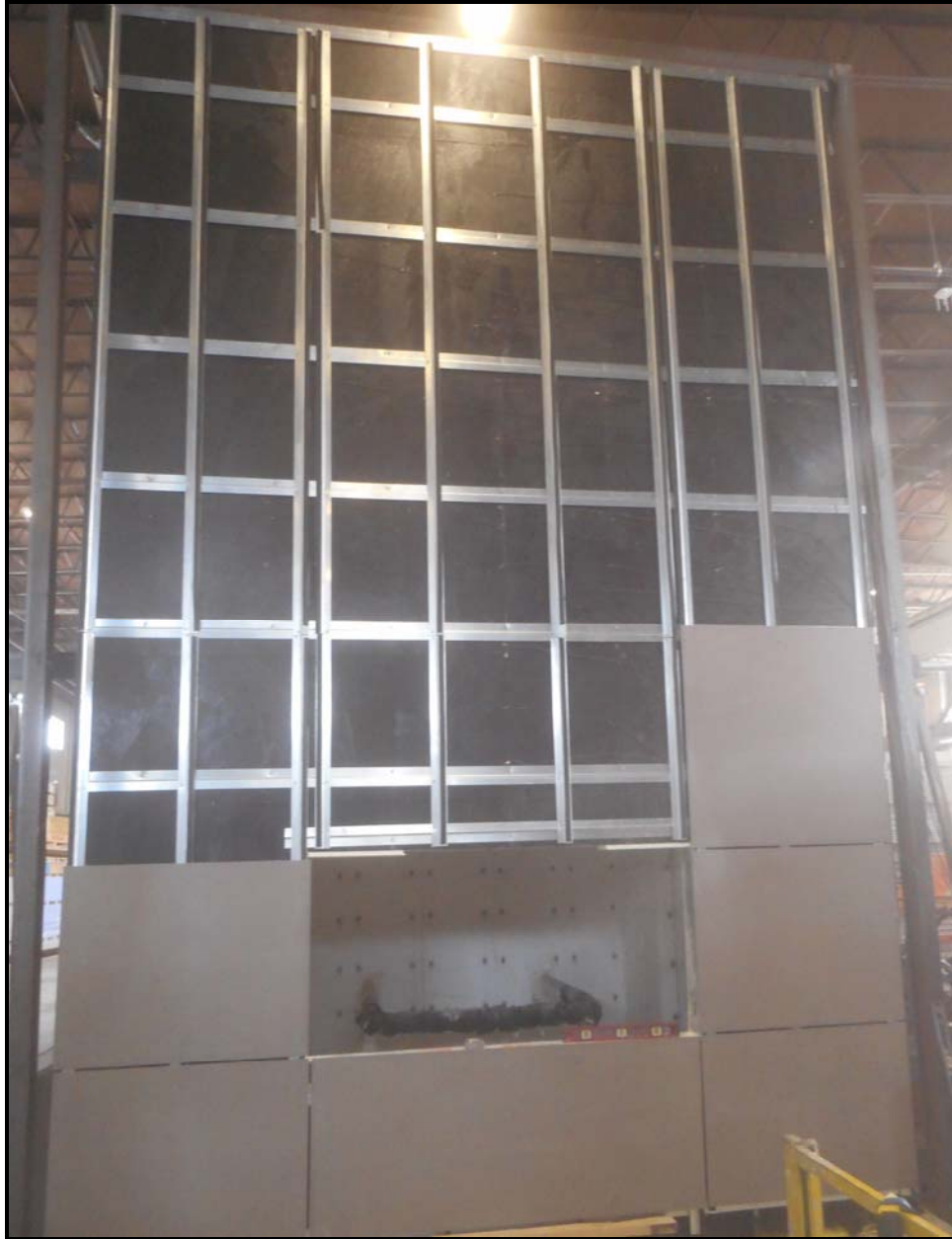
Photo 3: Horizontal and Vertical Z-Furring Strips and Start of SILBONIT Panel Installation
