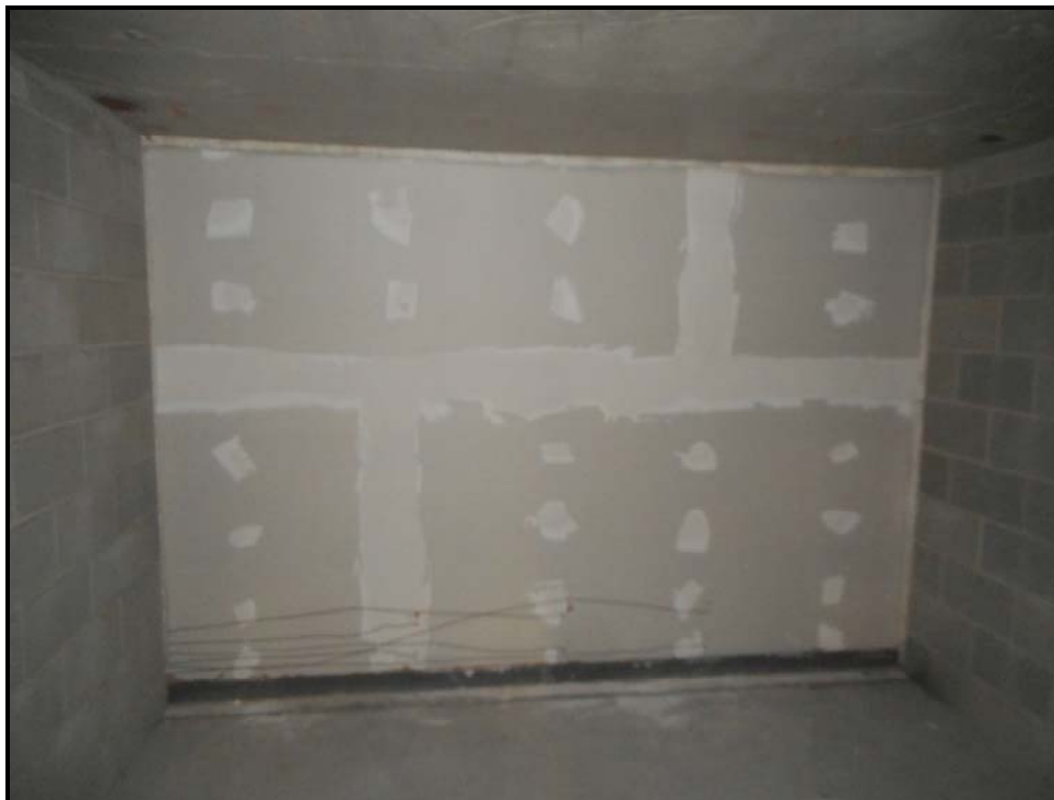
Photo 6: Complete Interior Second-Story Test Room
