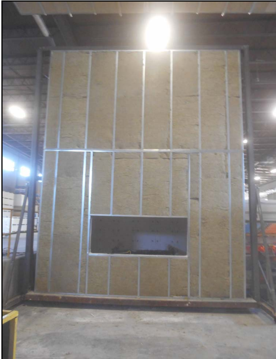
Photo 1: Core Wall Construction
