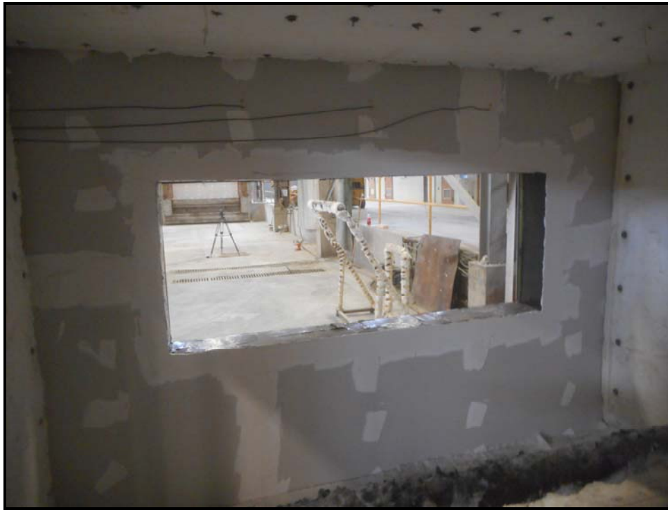
Photo 5: Complete Interior First-Story Test Room
