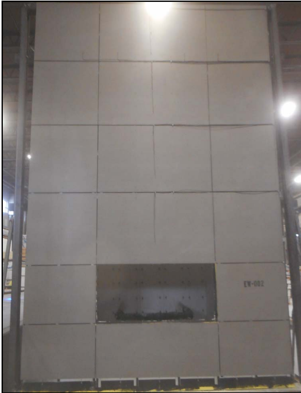
Photo 4: Complete SILBONIT Panel Installation
