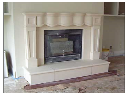
Raised Hearth Before Grouting
