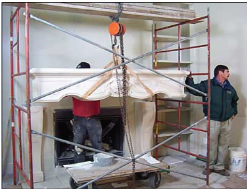
Lifting the Mantel Header
