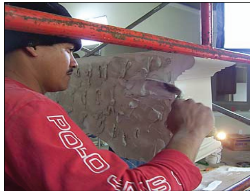
Applying Thinset Mortar to the Mantel Header
