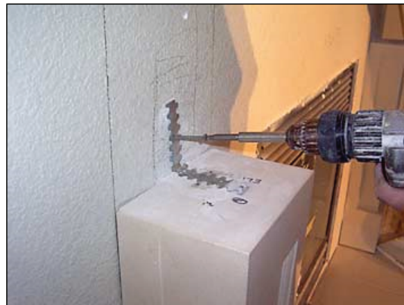
Attaching the Mantel Leg with a Masonry Tie
