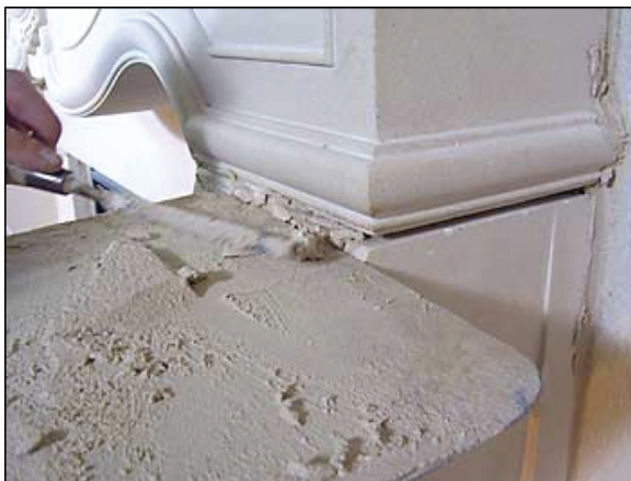
Applying Grout to the Mantel Joints
