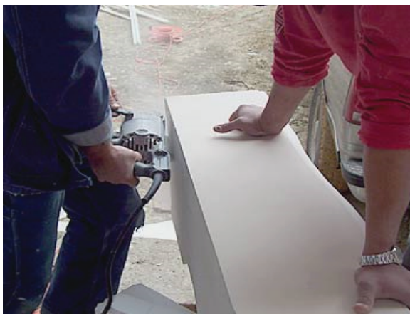
Cutting Slots to Match the Lag Screw Locations
