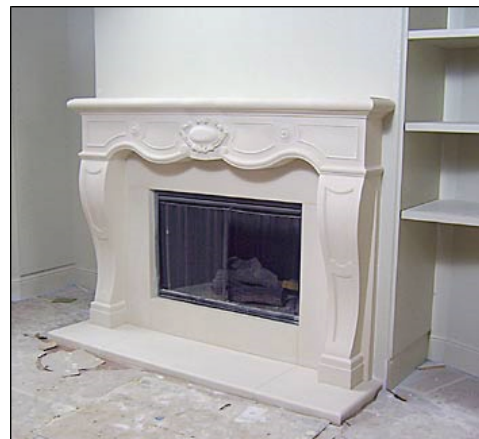
Finished Mantel Installation
