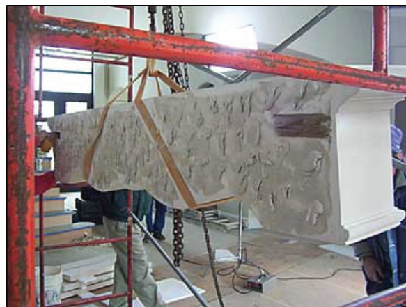
Setting the Mantel Header
