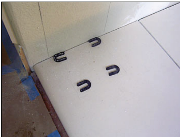
¼” Leg Spacer Placement
