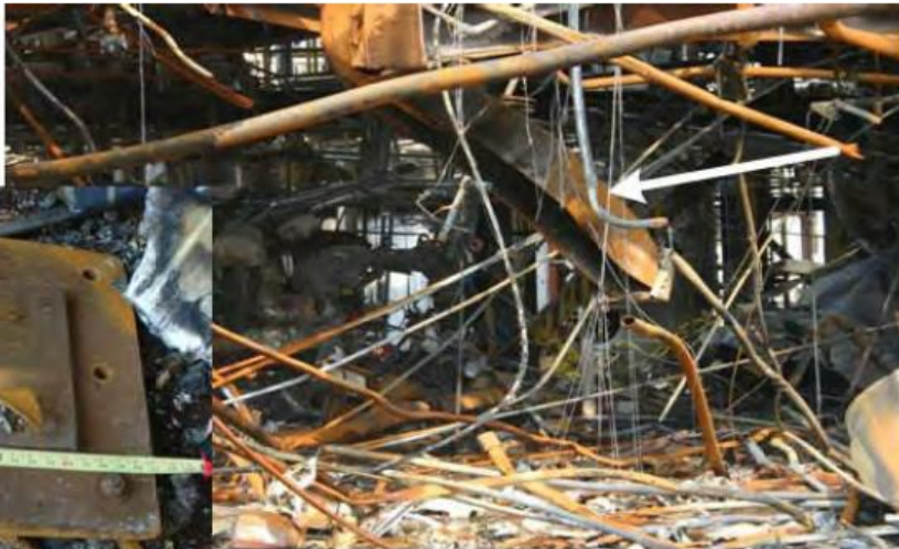
Support Column Sheared Off Baseplate
