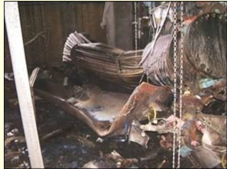
Heat Exchanger Rupture
