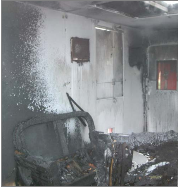
Figure 6.2.11(b) Clean Burn Pattern on Wallboard Behind Sofa.
