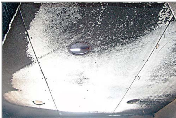
Figure 6.3.2.5(c) Pattern on Wall Created by Hose Stream.
