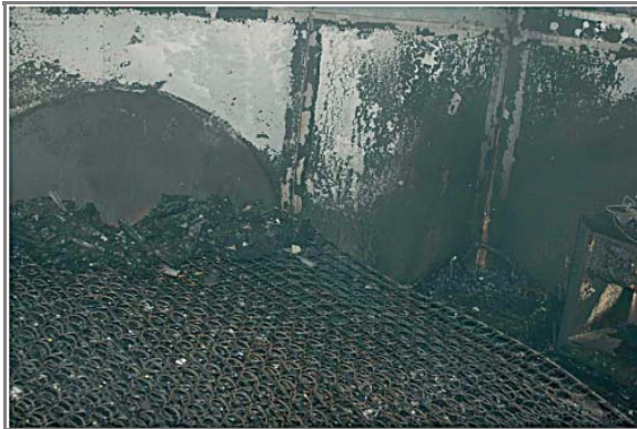
Figure 6.2.11.1 Clean Burn Above the Origin of a Test Fire.
