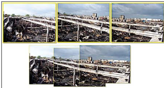
Figure 16.2.6.3 Three Individual Sequential Photographs of a Burned Wooden Pallet Factory (top), Made into a Physically Overlapped Mosaic (bottom).
