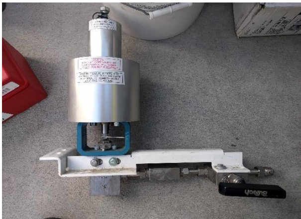
Figure 7: AOV 105 assembly fully removed
