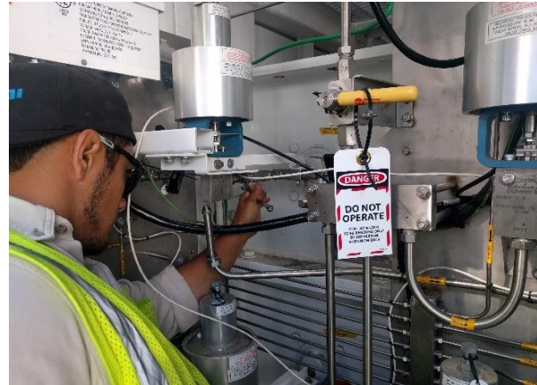
Figure 6: Remove all connections from AOV105 assembly
