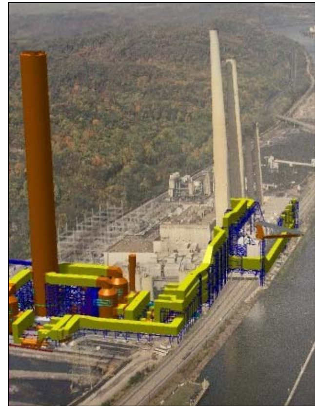
Sammis Plant with computer overlay of Wet Flue Gas Desulphurization (WFGD) equipment
