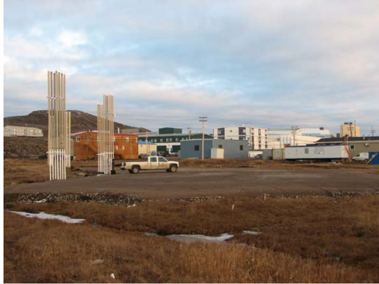
Figure 37. Foundation completed in fall of 2006, RCMP building, Iqaluit, NU
