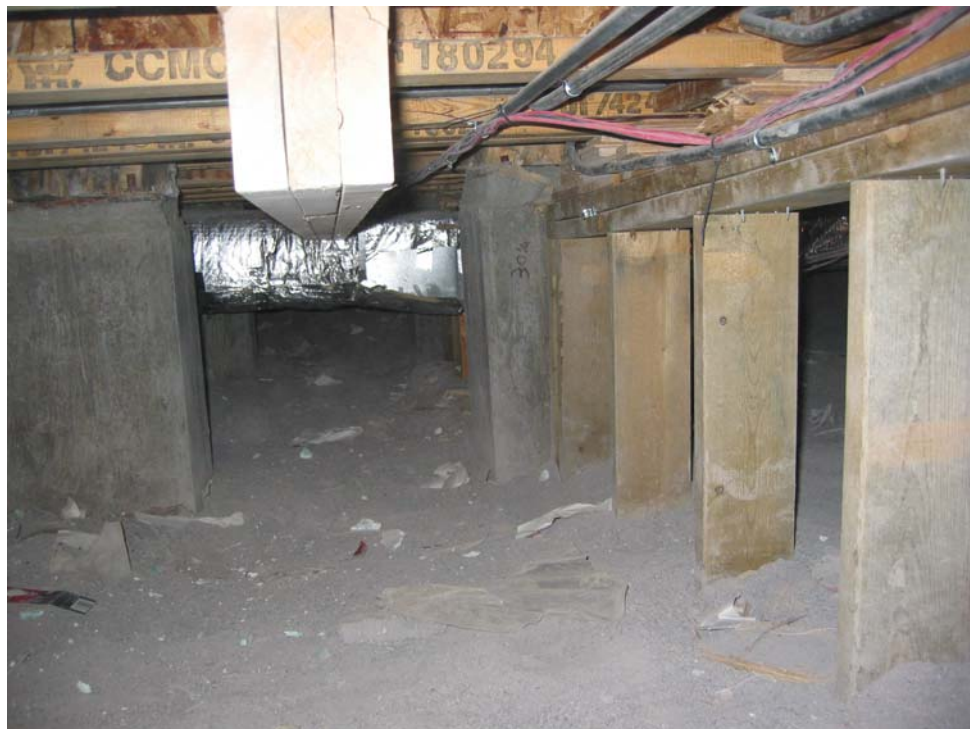
Figure A6. Photo showing concrete columns and wooden st resting on grade beams at Visitor Centre, Inuvik, NT
