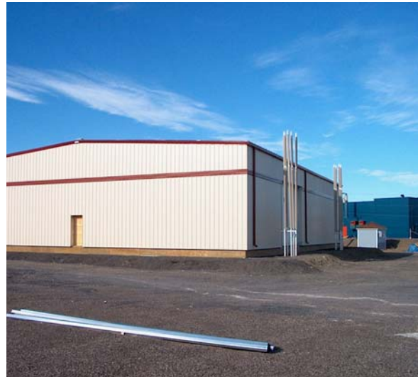
d) Flat Loop Thermosyphon Foundation – Airport maintenance garage, Inuvik, NT. (Courtesy AFC)
