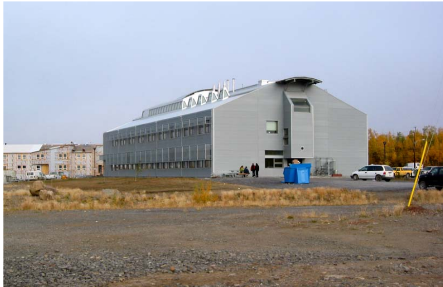
Figure 36. Aurora College, Inuvik, NT. Note: Good grade away from building.
