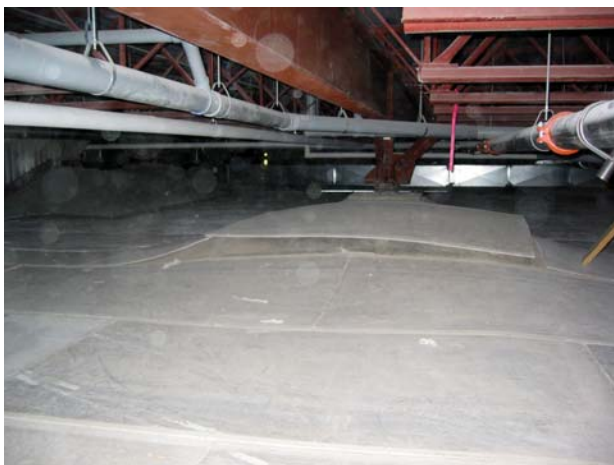
Figure 21. Services hung from floor girders at Inuvik Hospital
