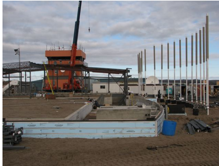
Figure 39. Kuujjuaq Air Terminal under construction, QC.
