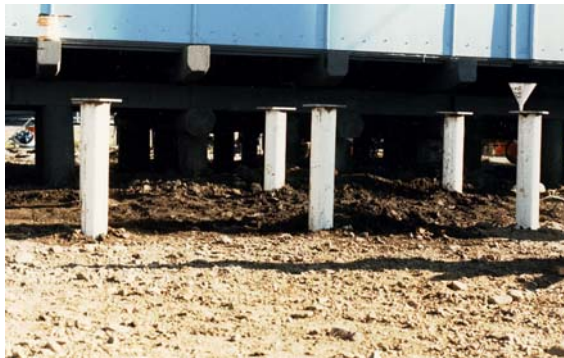
Photo 3. Slurry pipe pile foundation in Iqaluit, NU
