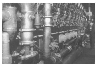
Flexmaster joints join water lines on a huge diesel engine.
