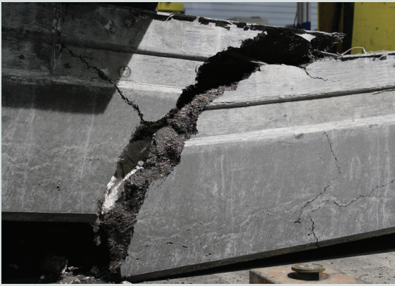
Figure 19. Close-up of failure in flexure.
