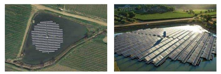
Figure 10: A-200 kWp grid-connected single axis based floating solar PV plant in Suvereto, Italy Source: Koine' Multimedia
