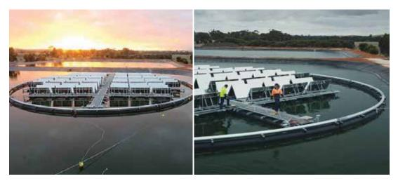
Figure 12: Phase I of 4MWp floating solar PV plant at wastewater treatment facility, Jamestown Australia Source: Infratech Industries
