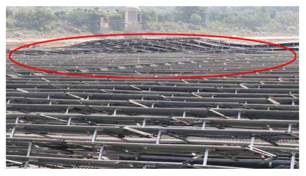
Figure 21: Impact of improper bathymetry and/or hydrography surveys
