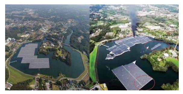
Figure 25: Japan's 13.7MWp floating solar PV plant before (A) and after (B). The red circle indicates that the anchoring and mooring line remained intact Source: KYOCERA (A) and PV Magazine (B)
