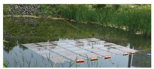
Figure 18: 0.57 kWp submerged floating solar PV based plant Source: MIRARCO mining innovation deployed in Sudhury, Canada
