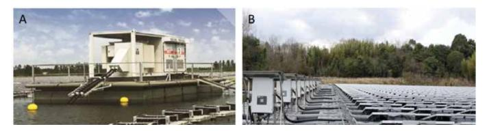
Figure 3: (A) Central inverter placed on floating platform at China. (B) String inverter Source: Sungrow
