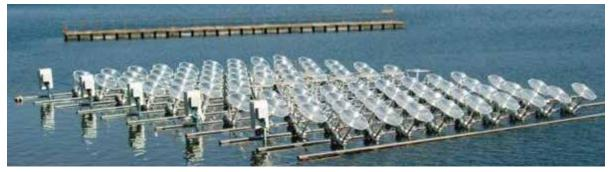
Figure 14: A pilot installation based on liquid solar array technology by Sunengy in hydro dam in India Source: Sunengy
