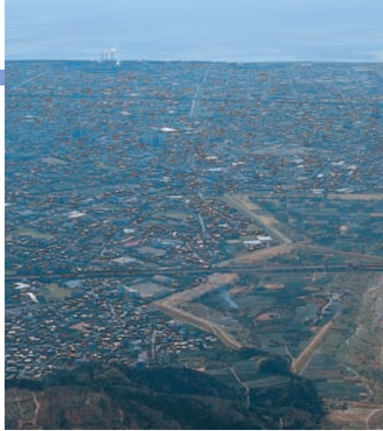
Karigane Embankment, resembling to Gecce flying in the sky, Fuji river mouth and Suruga bay.
