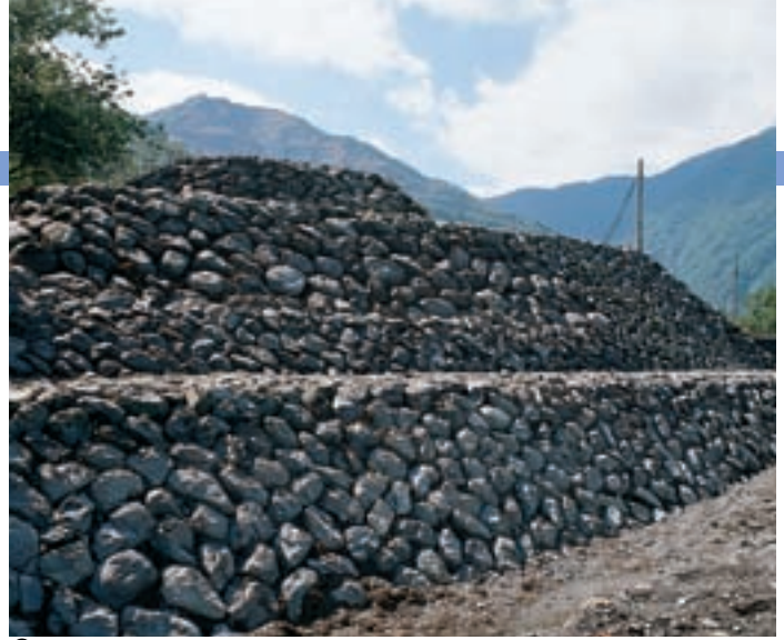
A Stone stack to control Midai river.
