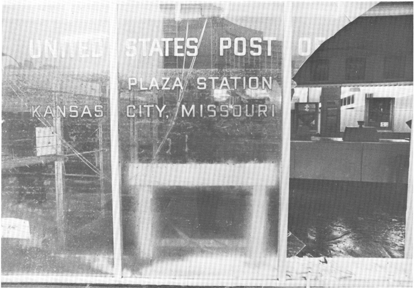
FIGURE 14.—United States Post Office, after Brush Creek flood crest, on Ward Parkway at Country Club Plaza, Kansas City, Mo.
