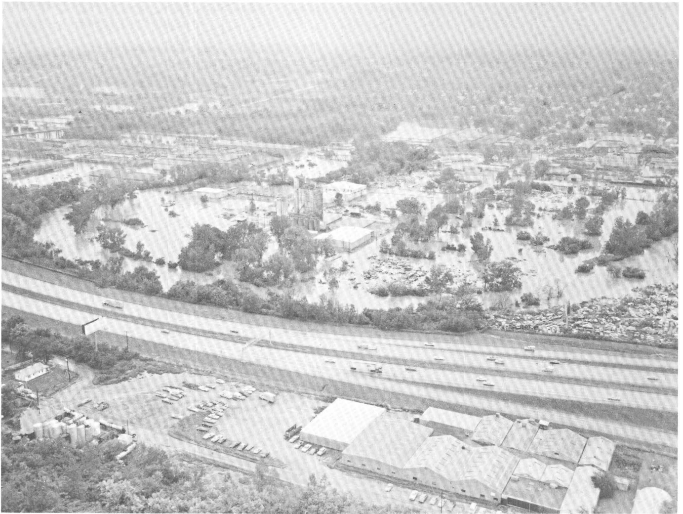
FIGURE 16.—Aerial view after flood crest, looking west along Blue River between 23rd Street and Truman Road, Kansas City, Mo.
