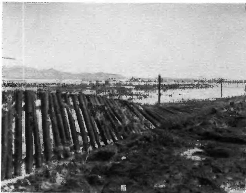
DAMAGE TO NORTHERN PACIFIC RAILWAY BRANCH LINE NEAR BREIEN.
