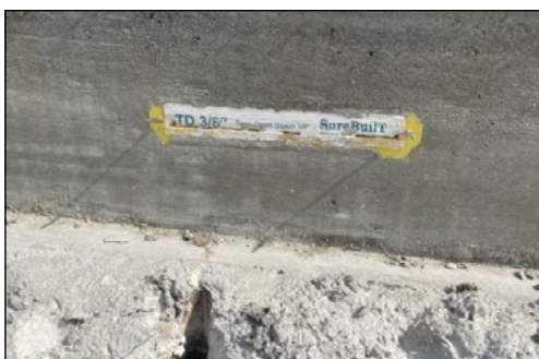
Dowels are inserted into sleeves after edge forms have been removed.
