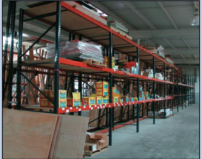
VIEW OF PALLET RACKING
