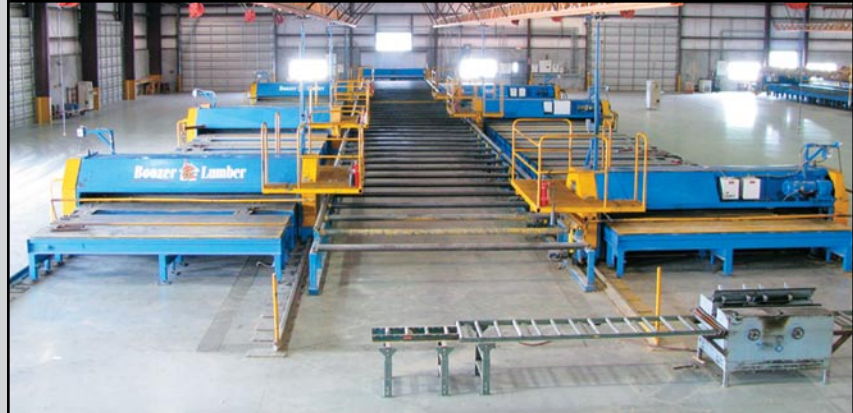
VIEW OF (2 OF 4) MITEK ROOF TRUSS LINES
