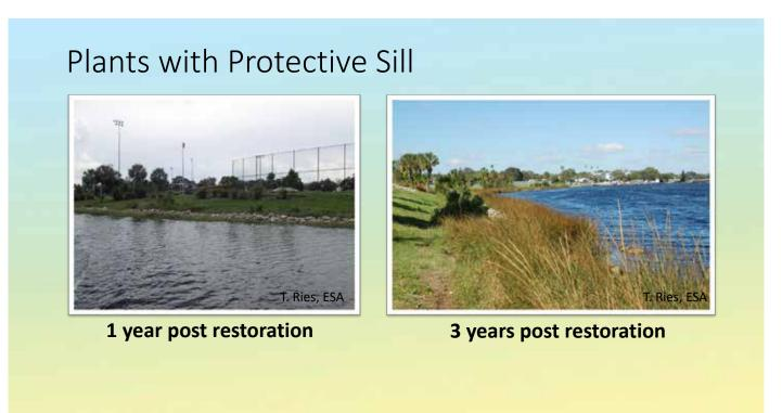
One year post restoration at Stewart Middle School (SMS) - left image and 3 years - right image, note that the rock sill is almost invisible (even though it runs the entire length of the (2,000') of the shoreline. This has been in the ground for over 10 years (2019) and in despite continual boat traffic (wakes), it has been stable and there is NO erosion along this bank!
