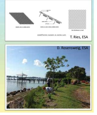
Geoweb<sup>®</sup> is a trademark name for a plastic accordion like material, typically 6" tall which can be expanded and anchored in place. These resultant cells can be filled with small rock or sediment and this matrix helps stabilize the ground. These can be used for vehicular wet crossings or planted with native vegetation for shoreline stabilization needs.
