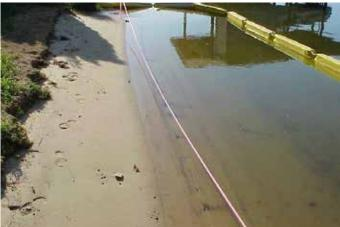
Figure 2. To qualify for a small-scale living shorelines permit exemption, the project must include plans to deploy a turbidity curtain to control silt and sediment. Credits: Rick O'Connor, Florida Sea Grant
