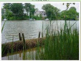
In areas with minimal wave energy; plantings with temporary protection, in the form of fiber-logs can provide temporary protection while the plants are growing/maturing; these work best in freshwater applications and can provide energy dissipation for up to 18 months, which should allow the plants the time necessary to coalesce. These applications do need initial monitoring and likely some maintenance to ensure that the plants are growing and expanding as anticipated!
