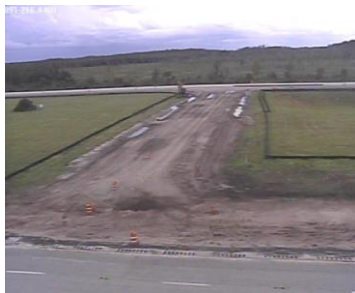
Under construction Aug 2013
