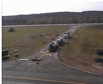
Nearing completion Nov 2013
