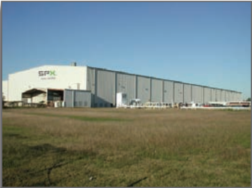
SPX Flow Control, Headquarters Houston, TX
