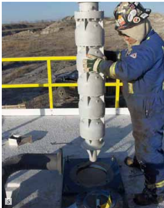
1: Installing two vertical turbine pumps in the field
