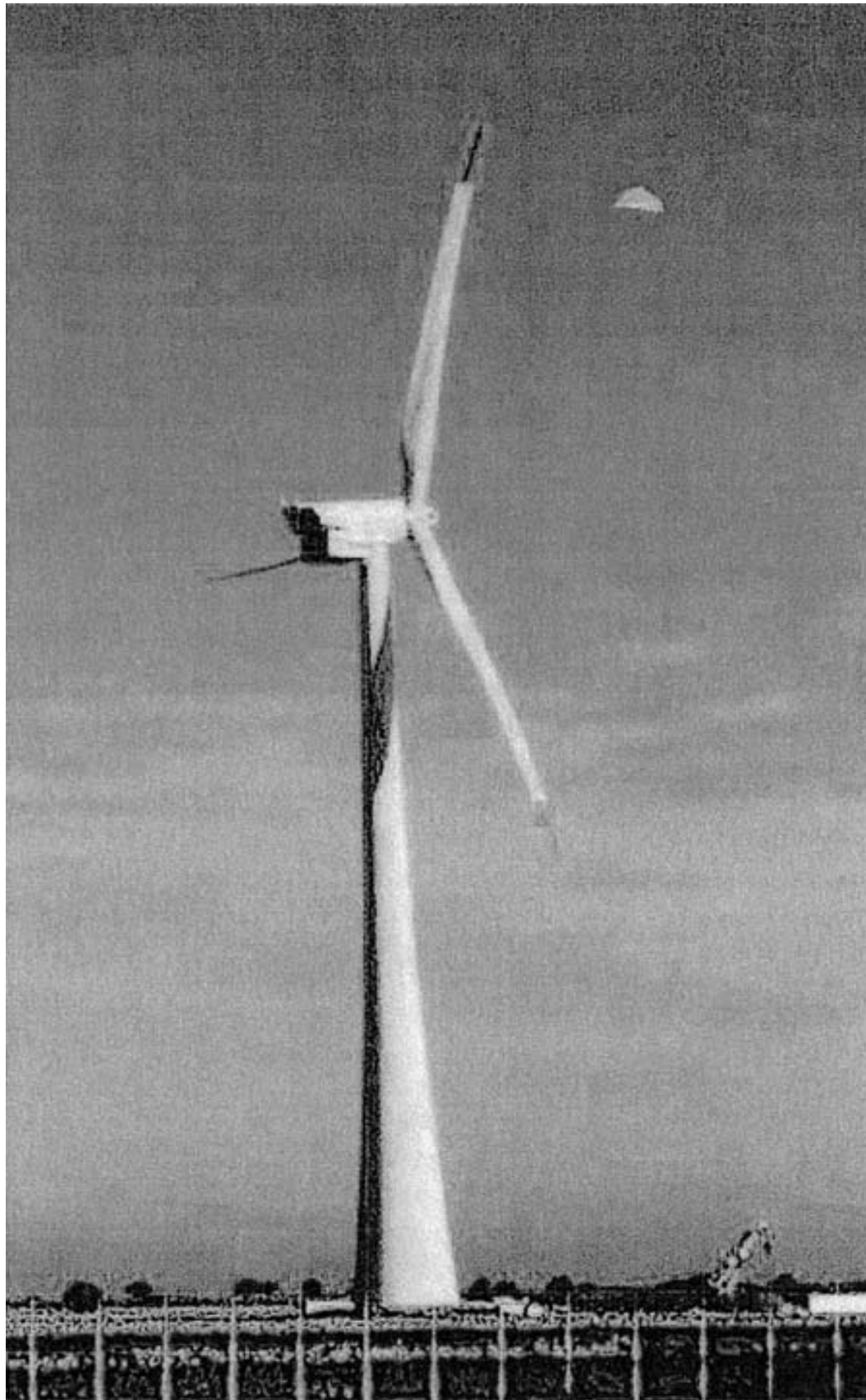
FIG. 10.4. (a) First General Electric baseline HAWT, 3.6 MW, 104 m diameter, operating at Barrax, Spain, since 2002. (Courtesy U.S. Department of Energy.)
