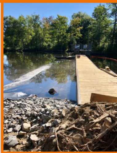
Construction at Long Pond
