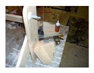
**5** - Push the bolt and tubing from the inside of part **D**. Then add the washer in between and push the assembled part **H&I** in place. Add the flat washer, then lock washer and tighten the nut. The tops of parts **D & H&I** should be flush and square. If not, sand both sides of the chair, so they are exactly the same height.
