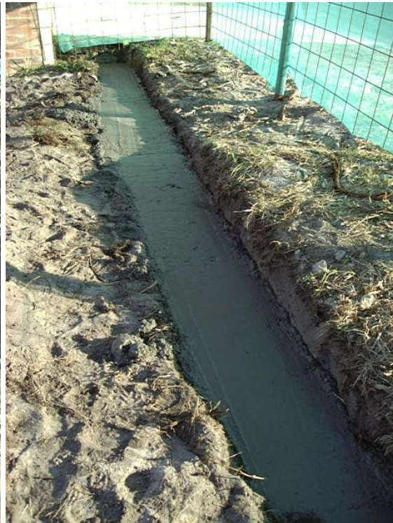
Strip footing after pouring of concrete
