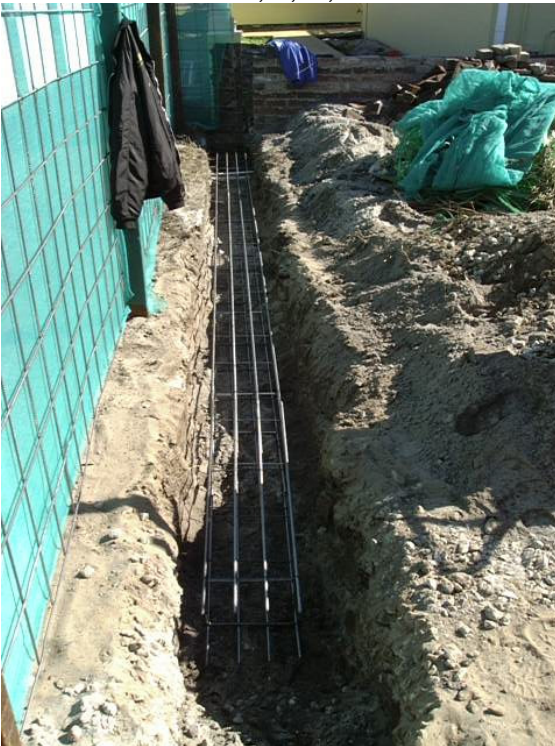
Strip footing trench with trench mesh reinforcement
