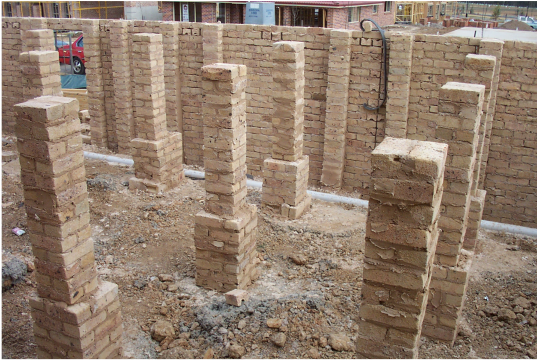
Isolated brick piers on pad footings
