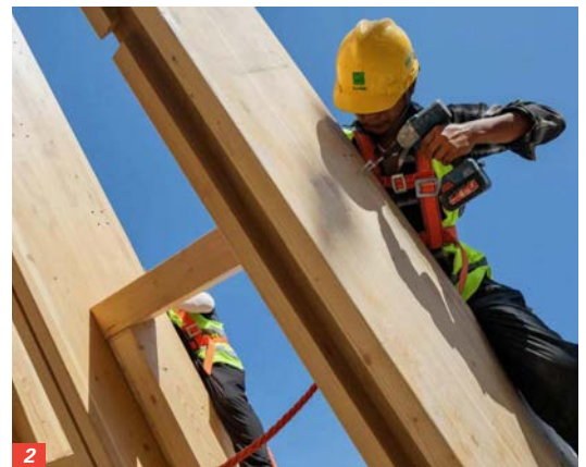
1/ A Skytrain station has been divided into east and west sides symmetrically arranged on top of the flyover. 2/ Douglas fir milled in Canada was used for the glulam components of China’s Olympic Sports project.
