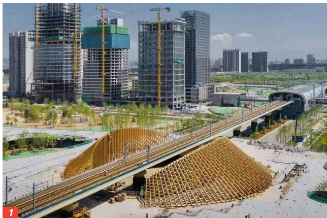
1/ A Skytrain station has been divided into east and west sides symmetrically arranged on top of the flyover. 2/ Douglas fir milled in Canada was used for the glulam components of China’s Olympic Sports project.
