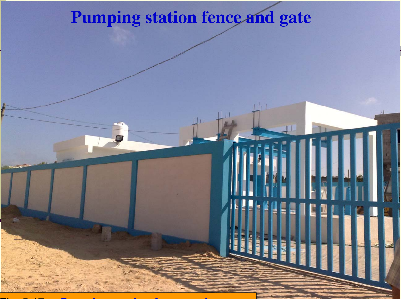
Fig. 5.17 Pumping station fence and gate
