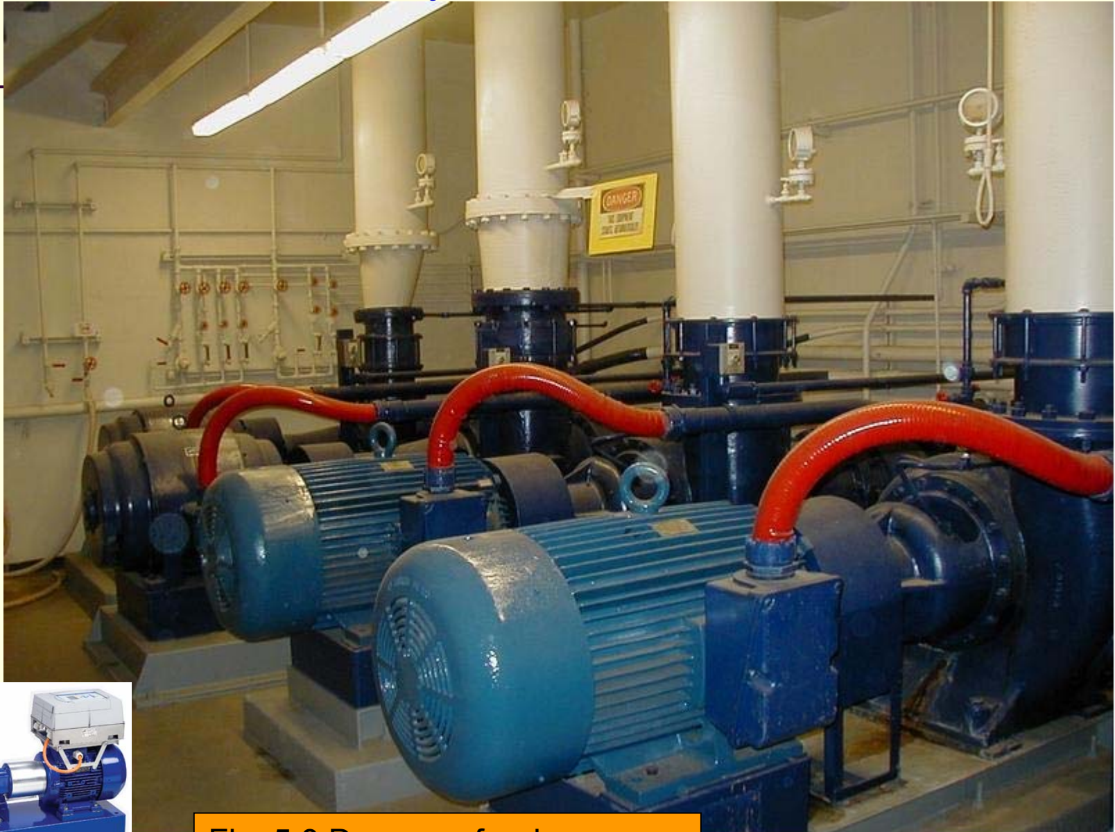
Fig. 5.8 Dry room for dry pumps
