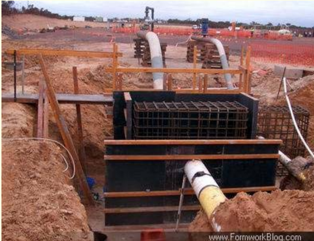
Fig. 5.33 Thrust block under construction
