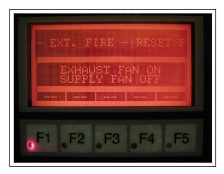
FIGURE 22-1 DISPLAY PANEL EXTERNAL FIRE CONDITION
