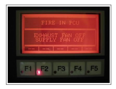
FIGURE 21-1 DISPLAY PANEL FIRE IN THE PCU CONDITION
