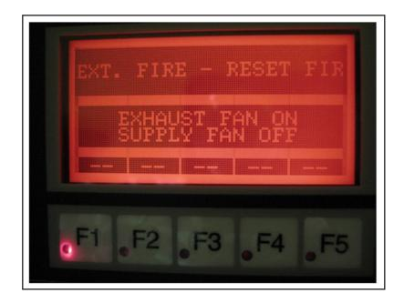
FIGURE 23-1 DISPLAY PANEL EXTERNAL FIRE CONDITION RESET SYSTEM
