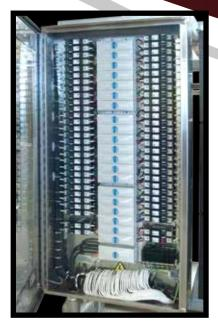
**Power Distribution with Sealed Breakers**
