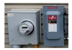
Switching this disconnect OFF will cause the entire system to power down immediately.
