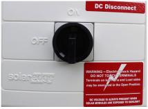
Switching this disconnect OFF will cause the connection between that inverter and the array to be turned off immediately.
