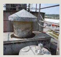
SITRANS LR560 measure the level of malted barley at United Canada Malt Ltd The compact size of SITRANS LR560 is easy to carry to the top of the silo.
