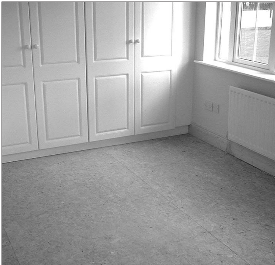
Sophisticated forest products such as oriented strand board (OSB), shown here in a flooring application, are now being manufactured in Ireland from Irish wood.
