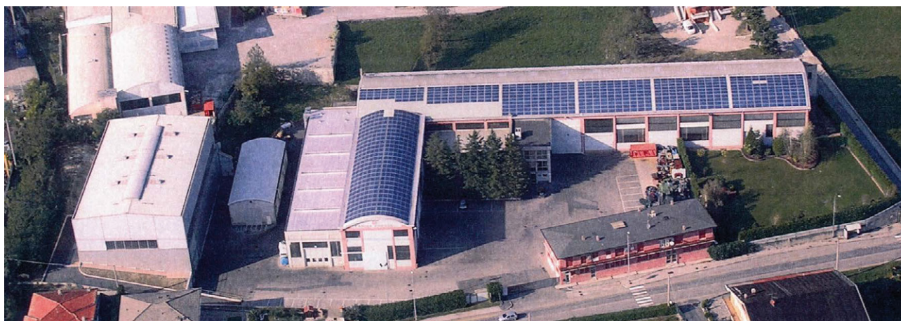
Factory building in Suello (Lecco), Italy
