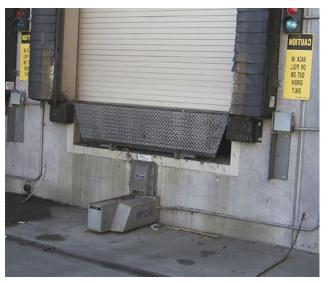
Dock mounted vehicle restraint clamps to a bar under the truck.
