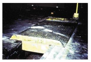
A projection below the surface prevents the dock board from shifting off its support.
