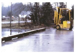
A bull rail at an unused edge of a dock reduces the risk of a forklift wheel slipping off.
