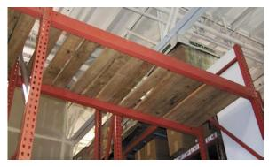
Check that wood stringers or decking in racks are in good condition. They may support the load if the pallet is not properly placed on both front and rear rails.
