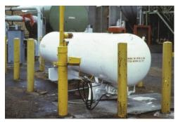
Propane tank used to refill the forklift LPG tank is protected against vehicle damage by heavy posts.
