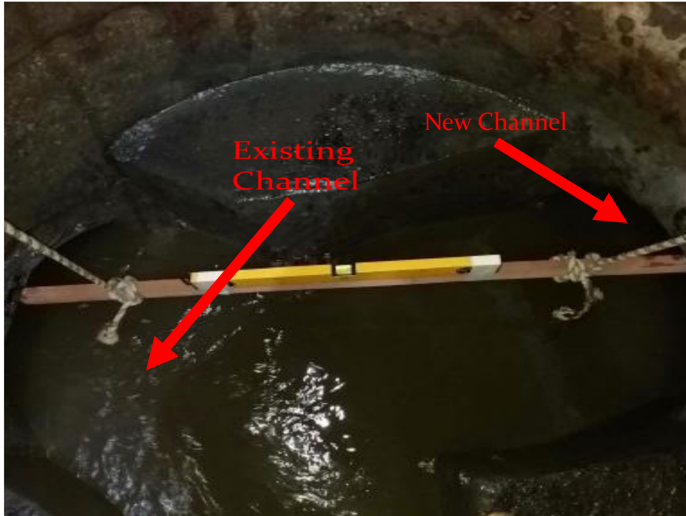
Soffit to soffit connection
