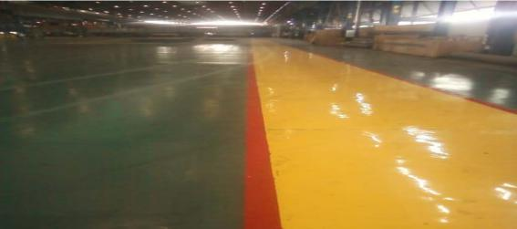
**12.Vaccum Dewatering System :** Providing Vaccum Dewatering System by using Tremix Flooring System For RCC floors and Roads
