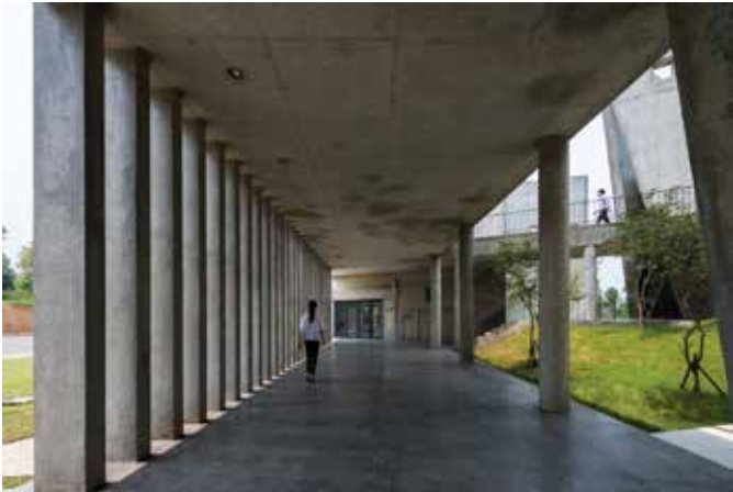
Fig. 8: A single-story open corridor connecting V-shaped buildings at the Viettel Offsite Studio
