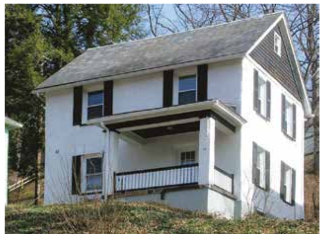
Fig. 9: Typical hollow-wall concrete house built in 1920 in Southmont, PA (near Johnstown) 16 (photo courtesy of Lu Donnelly/Western Pennsylvania History)
