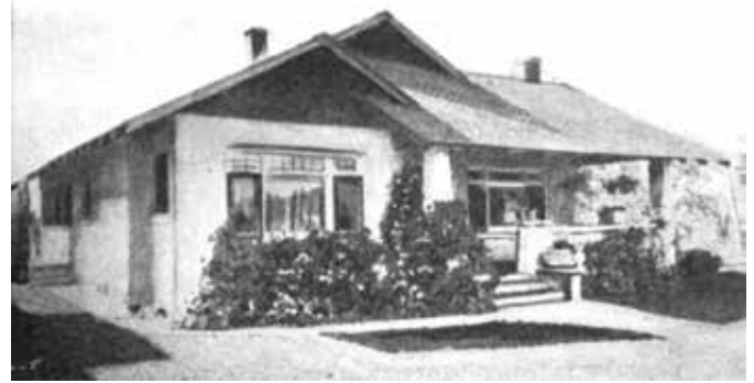
Fig. 5: Concrete hollow-wall bungalow built by W.H. Riley in Riverside, CA 10
