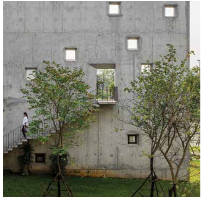
Fig. 7: Stepped square cutouts in the slabs allow some direct sunlight to pass onto the courtyards created by the V-shaped units
