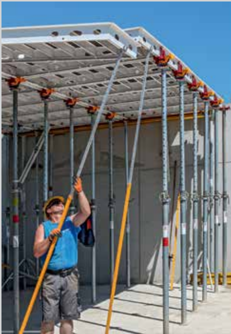
(photo courtesy of PERI GmbH)
