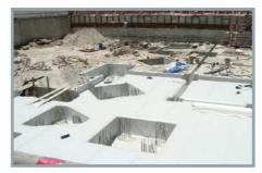
**Proofex PGP / Alkorplan**, a loose-laid PVC The **Nitoproof** liquid-applied coatings range membrane system, is available in large rolls. Joining is realised through welding with hot air. Compartments can be laid out using Supercast PVC waterstops which are welded to the membrane.
