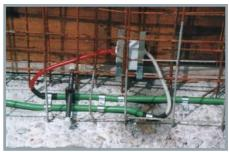
Supercast Predimax injection waterstops for future provision of sealing leaking joints.
