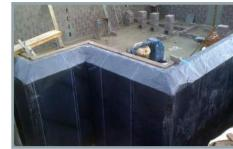
Post-applied bitumen based waterproofing for floors and walls can be easily installed using Proofex GP / 3000 self-adhesive membranes in conjunction with **Proofex** Protection Boards. Proofex 3000MR is ideal where gas is present in the ground or the soil is contaminated. The aluminium foil layer in the membrane provides resistance and long term durability.
