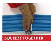
PVC waterstops should always be joined by welding using the process above, never by lapping. Fosroc supply jigs and heating blades suitable for making simple butt joints on site.
