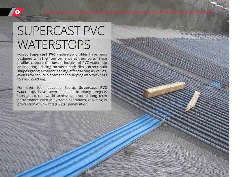
To ensure a firm fix, Fosroc Supercast Watafoil and Hydrofoil PVC waterstops incorporate a row of eyelets along both edges for wiring to nearby steel reinforcement.
