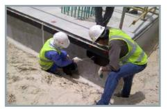
provides protection for foundations or for dampproofing, they are easy to apply and are available in a wide range of grades.
