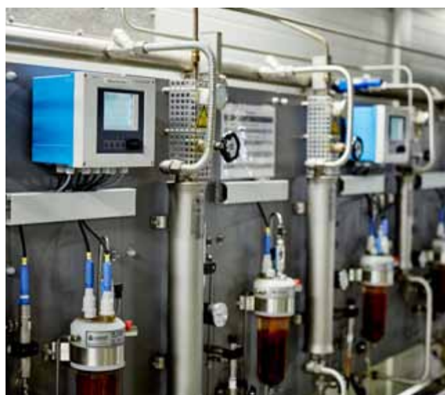
Sampling & analysis system - SWAS panel solution with analytical instruments: pH, conductivity, O 2 and silica
