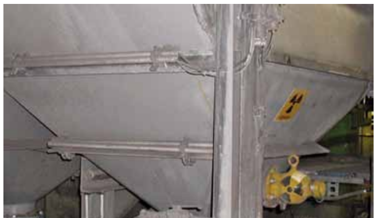
Gammapiilot - nuclear solution with its advantage of being mounted external to the hopper, away from the heat and abrasive ash
