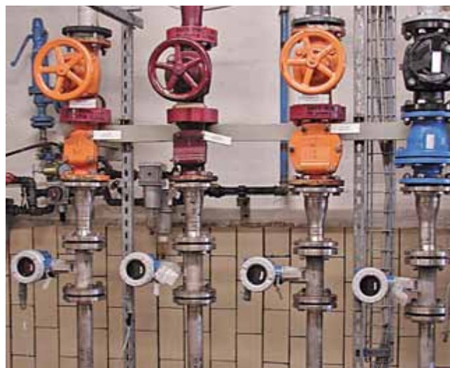
Prowirl monitors the volume flow of the fully demineralized water
