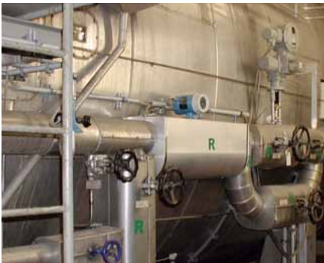
Promass compact version: due to the preheated oil, the pipes are isolated
