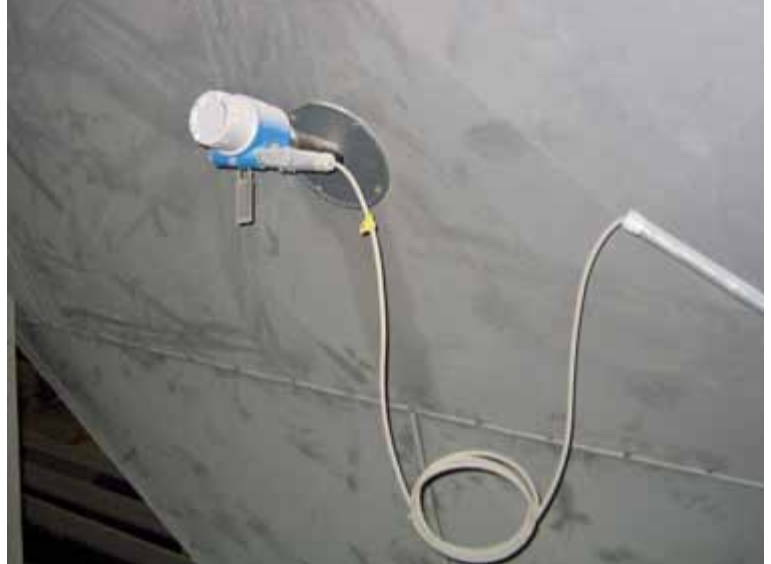
Capacitance switch for high level fly ash indication inserted through the hopper wall at the point where indication is required
