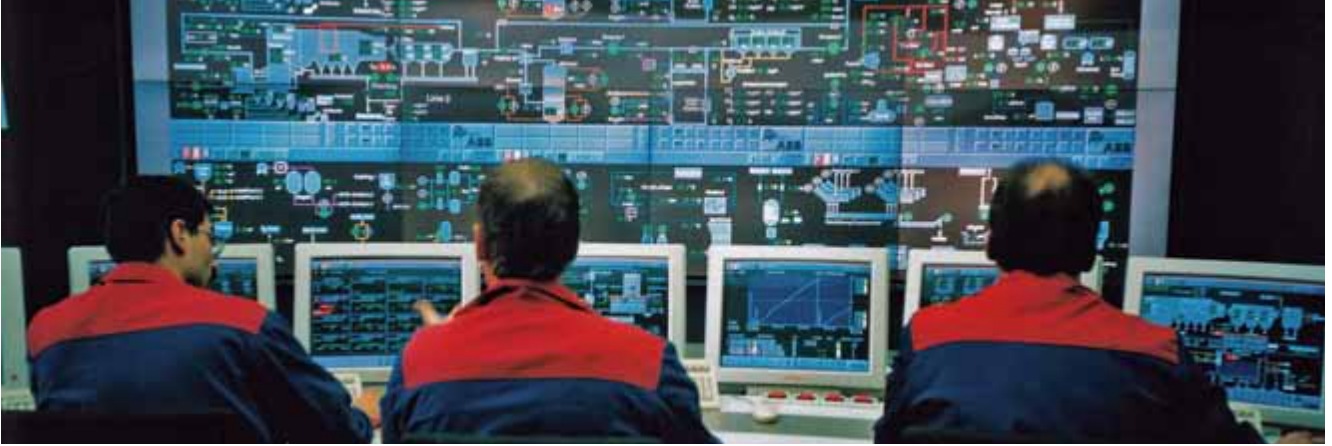
Control room of a modern power plant
