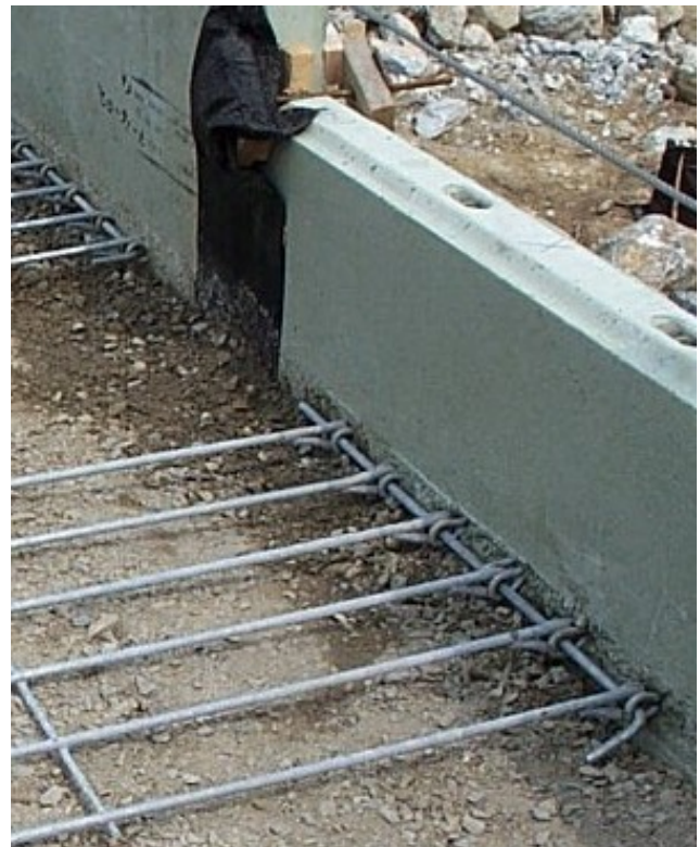
Figure 5: Reinforcement Mesh Attachment to Panel
