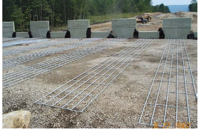
Figure 1: Steel Mesh being placed in layers of compacted fill.
