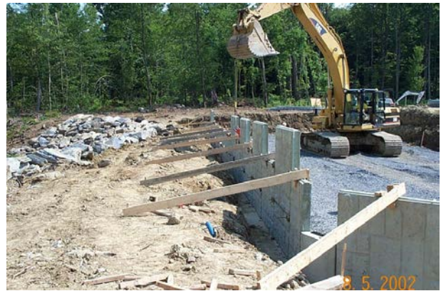
Figure 4: Placement of first row of panels
