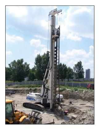
Figure 6-1. Short Flight Auger.
