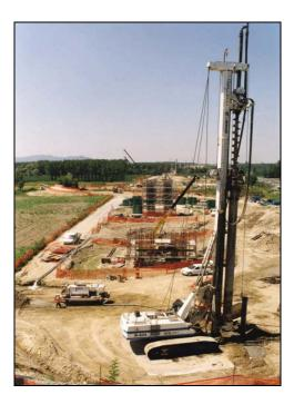
Figure 6-14. Crawler Mounted Drill Rig.
