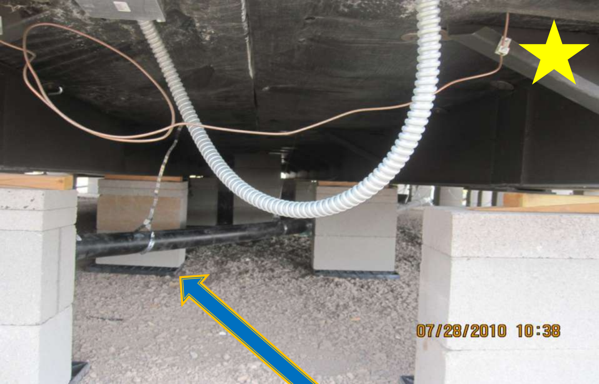
Plastic pads are inverted for CMU block use
