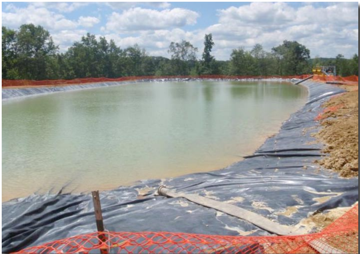
Figure 15: Typical lined freshwater pit for water storage before fracking operation. Photo courtesy of ALL Consulting, http://www.netl.doe.gov/technologies/oil-gas/publications/epereports/shale_gas_primer_2009.pdf
