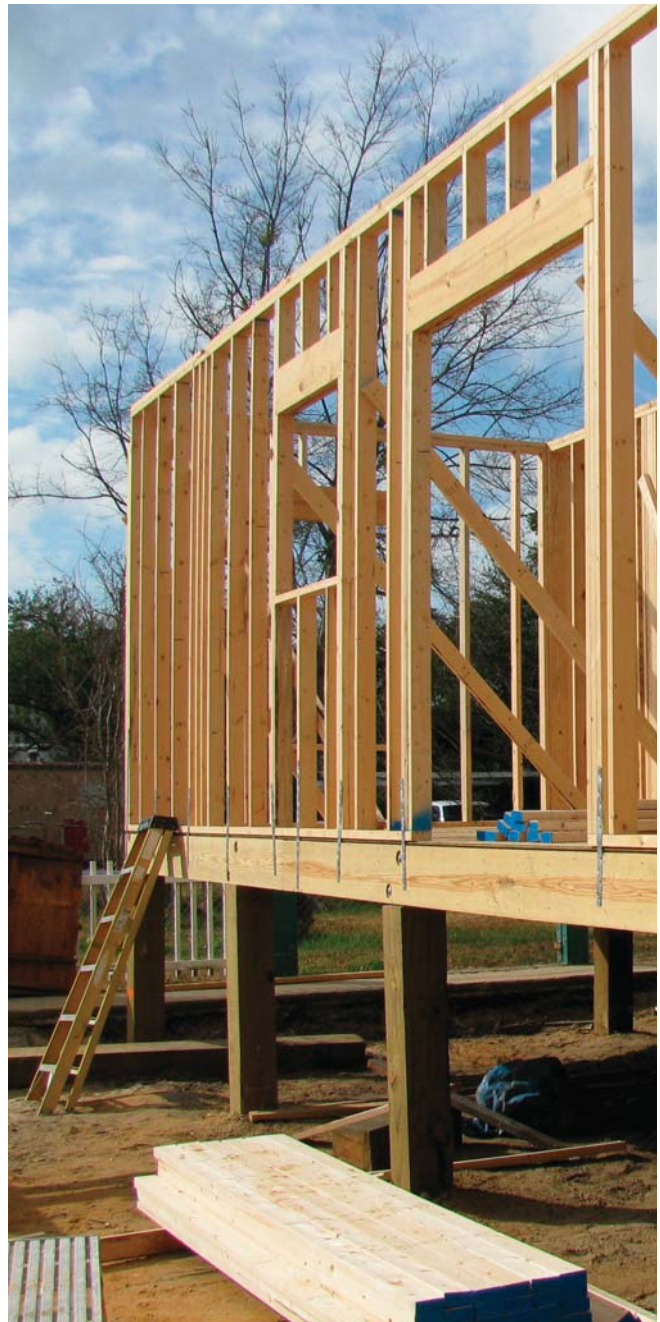
(Fig. 1) A wall and doorway are shown framed in at a house on Mississippi's Gulf Coast
