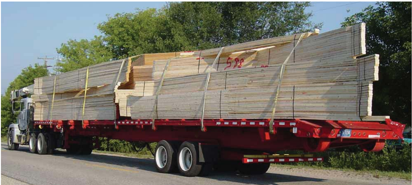
(Fig. 28) Similar to other dimensional building systems, trusses are delivered from the builder in packages according to specification.
