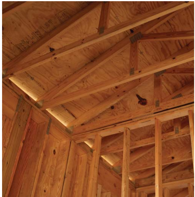
(Fig. 26) Wood roof trusses sit on an exterior bearing wall.
