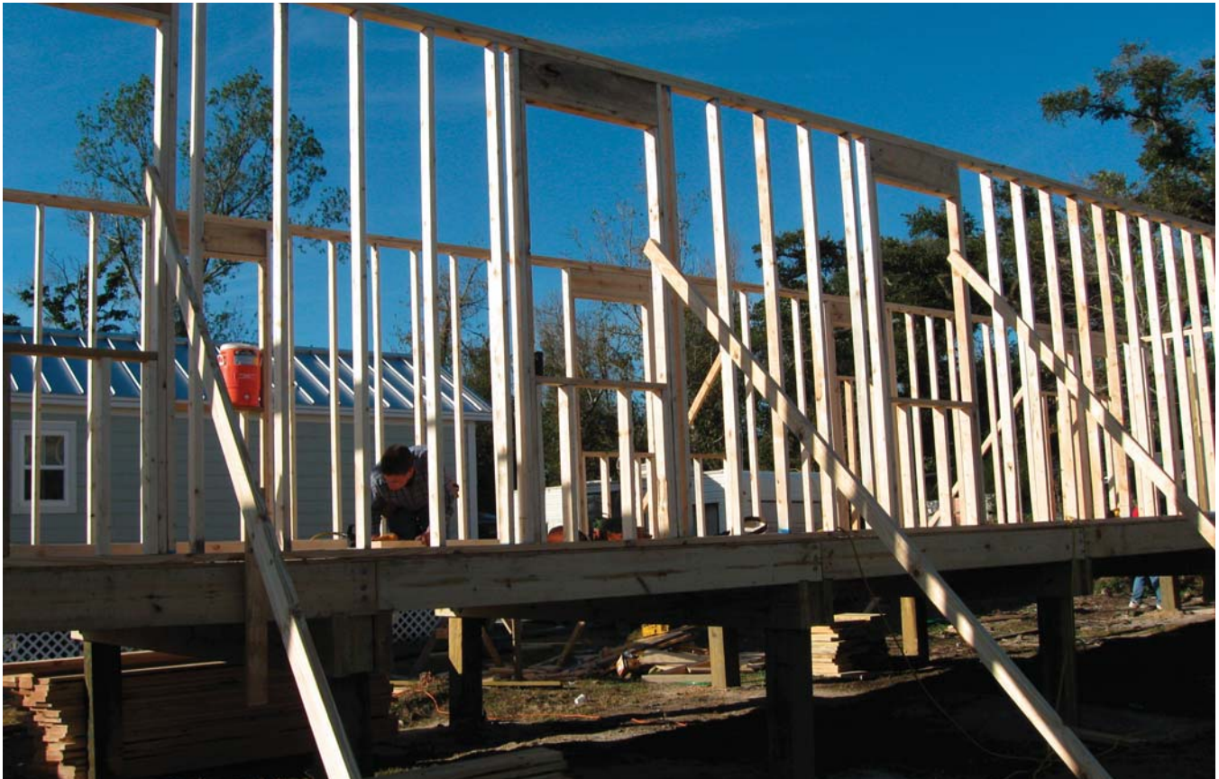
(Fig. 5) Exterior walls are held plumb by bracing until interior walls are framed.
