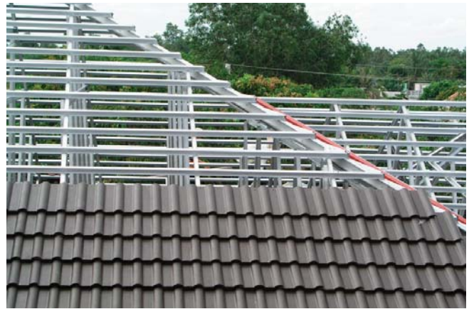
(Fig. 24) Lightweight steel trusses allow for design flexibility and are resistant to corrosion.
