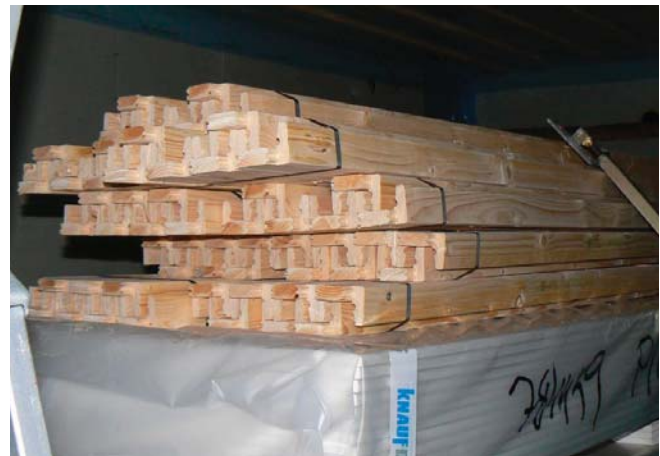
(Fig. 11) Finger jointed i-beam engineered studs arriving on-site in a lumber package delivery.
