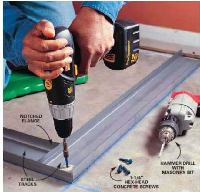
(Fig. 13) Steel stud walls are constructed with upper and lower guide tracks that are attached to the ceiling and floor.
