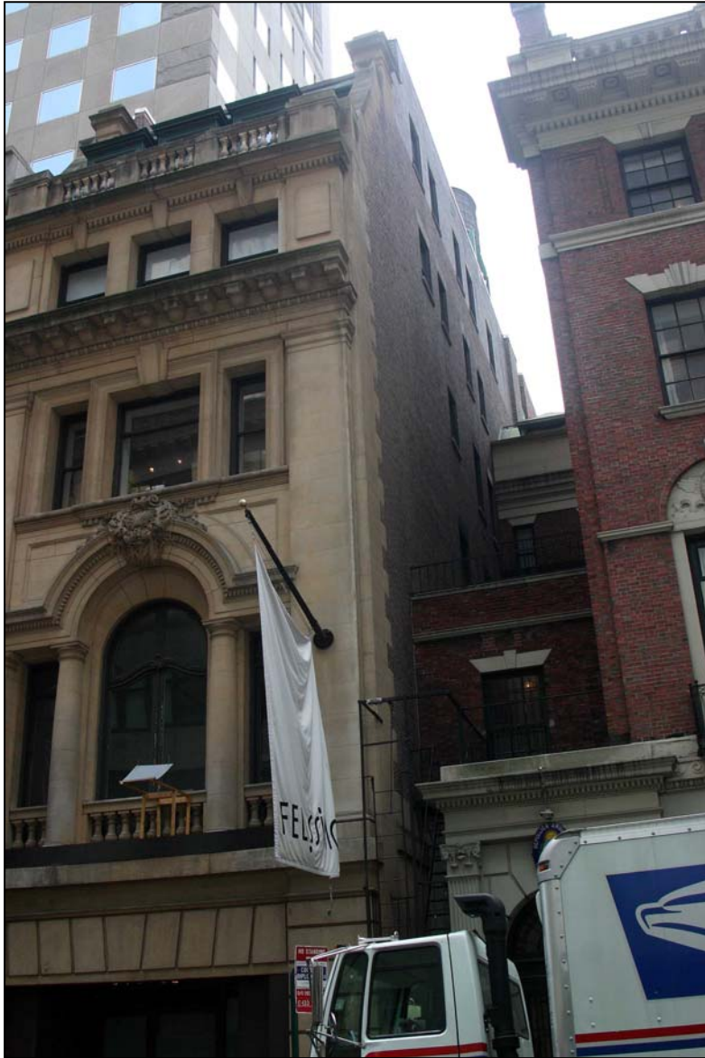
10 W. 56 th Street West Elevation
