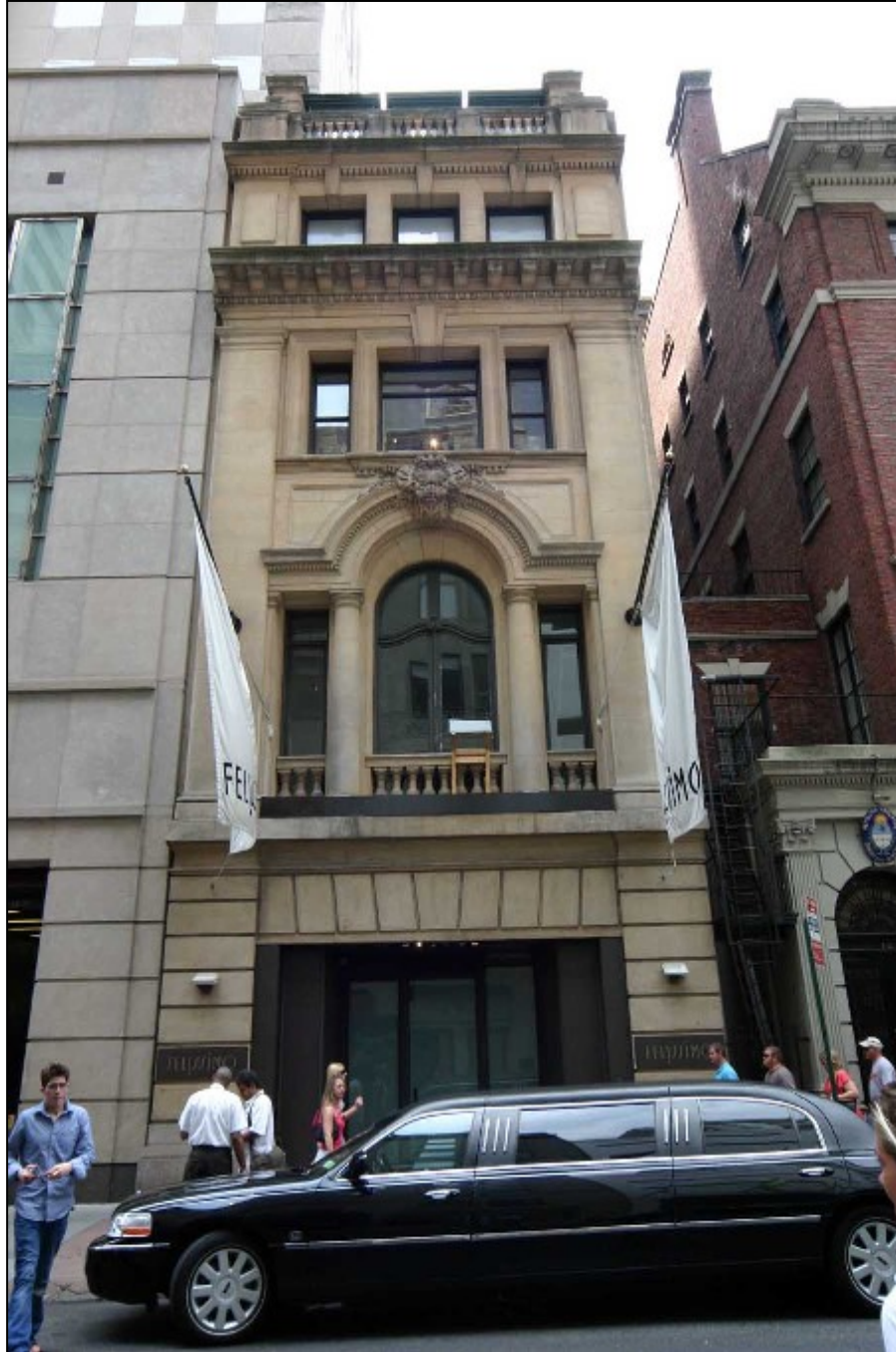
10 w. 56 th Street -- South Elevation
